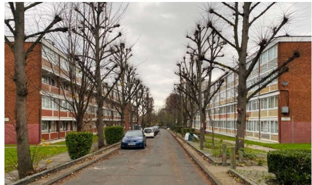
Figure 1. Alton Estate, Harbridge Avenue, Four Storey Maisonettes
